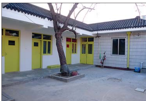
HomeShop is a courtyard house that has individual studio rooms and one larger co-working space with desks and wireless Internet.
